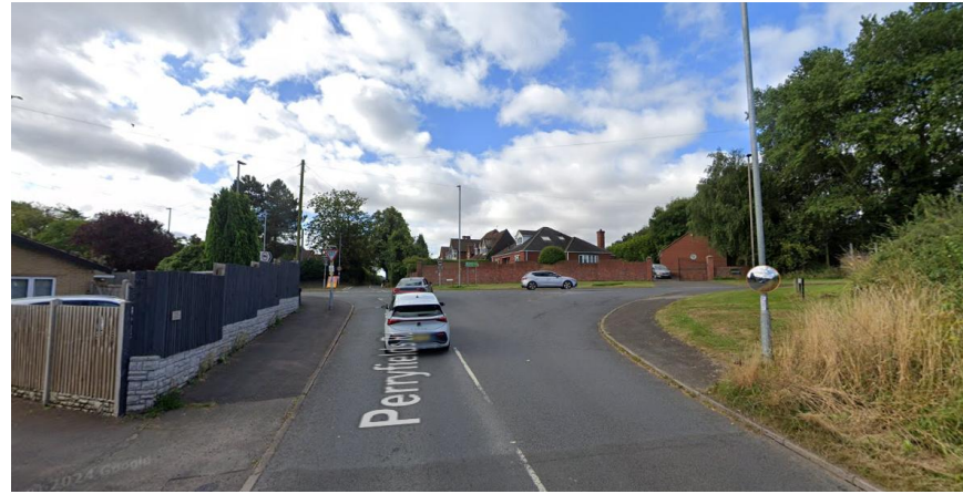
StreetView along Perryfields Road looking south
